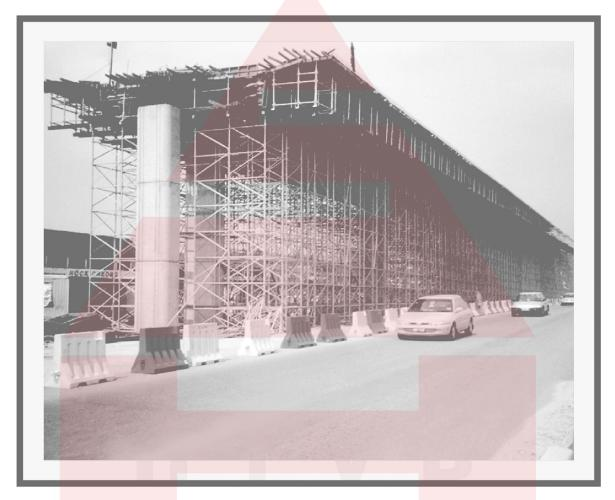
Huatraco® C60 Shoring System is a multi-directional & multi-level heavy duty shoring equipment to support all types of heavy structures, and is manufactured to comply with British Standard BS 5975 and BS EN 12812.
