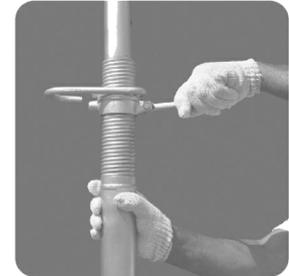
Adjust the height by sliding the screw position.
